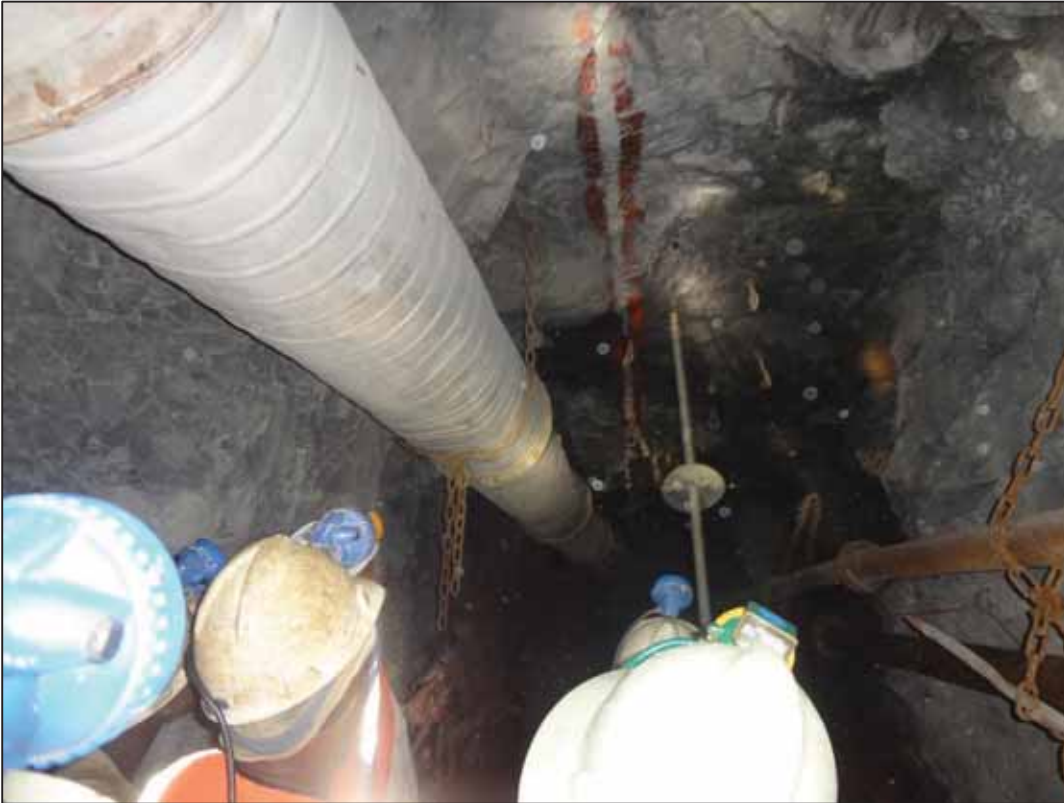
Figure 68: Development excavation greater than 2m high with poor hanging wall conditions and overhanging side wall (Mining House D)
