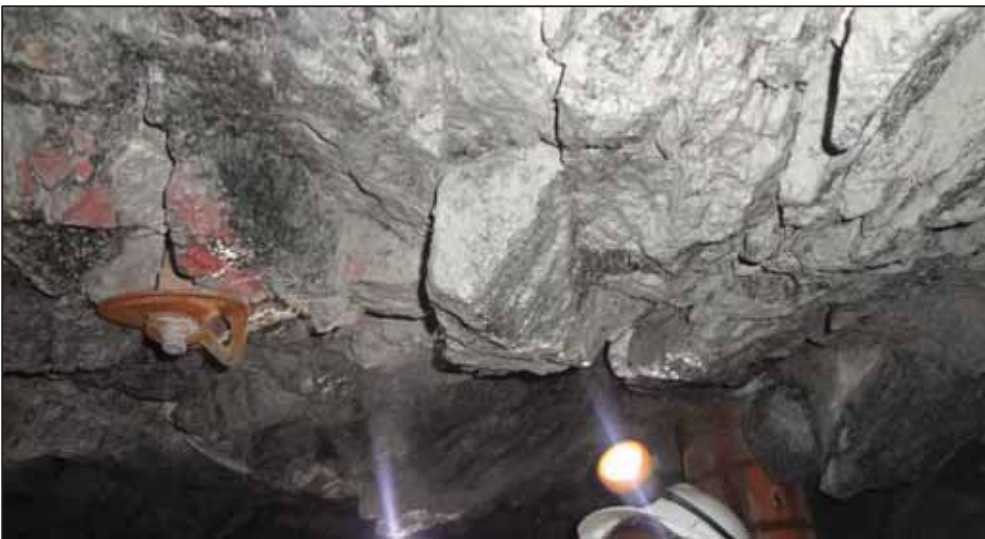
Figure 25: Prominent Hanging Wall Jointing (Mine 10)
