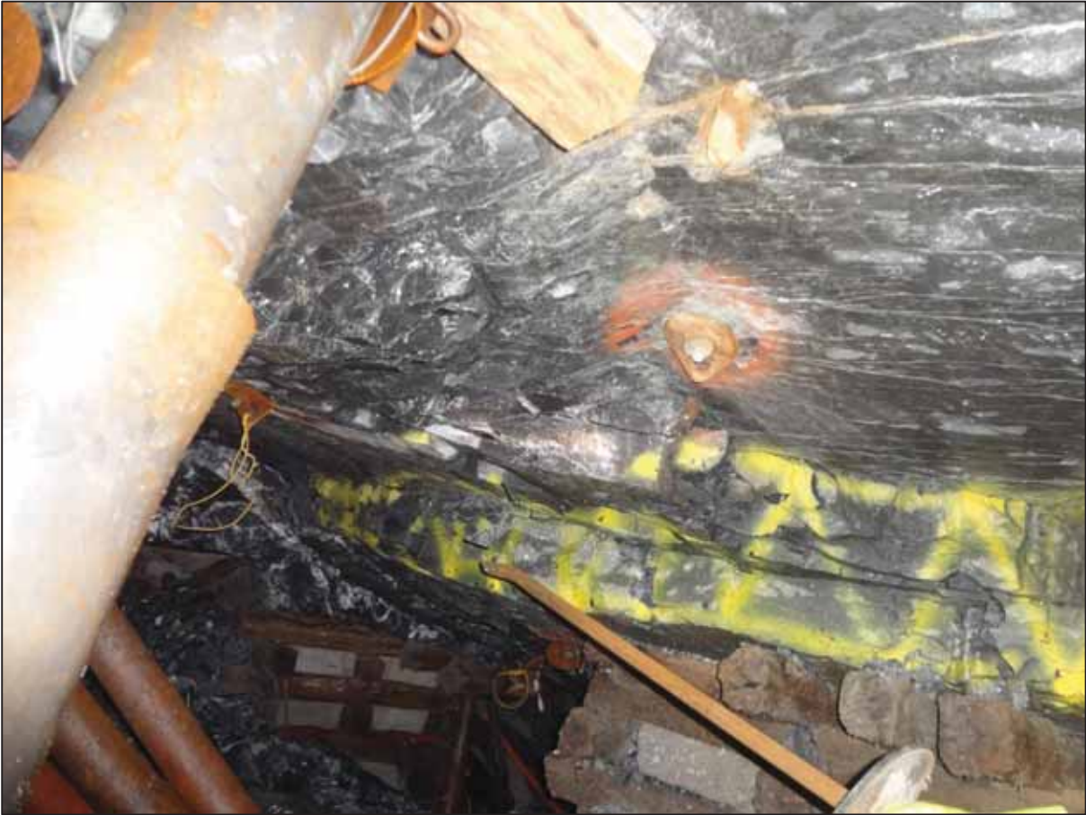
Figure 63: Layering and fractures in lava hanging wall (Mine 8)
