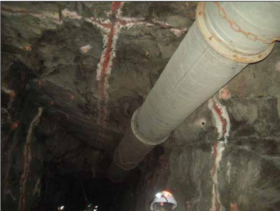
Figure 28: Development excavation greater than 2m high with poor hanging wall conditions and overhanging side wall (Mine 9)
