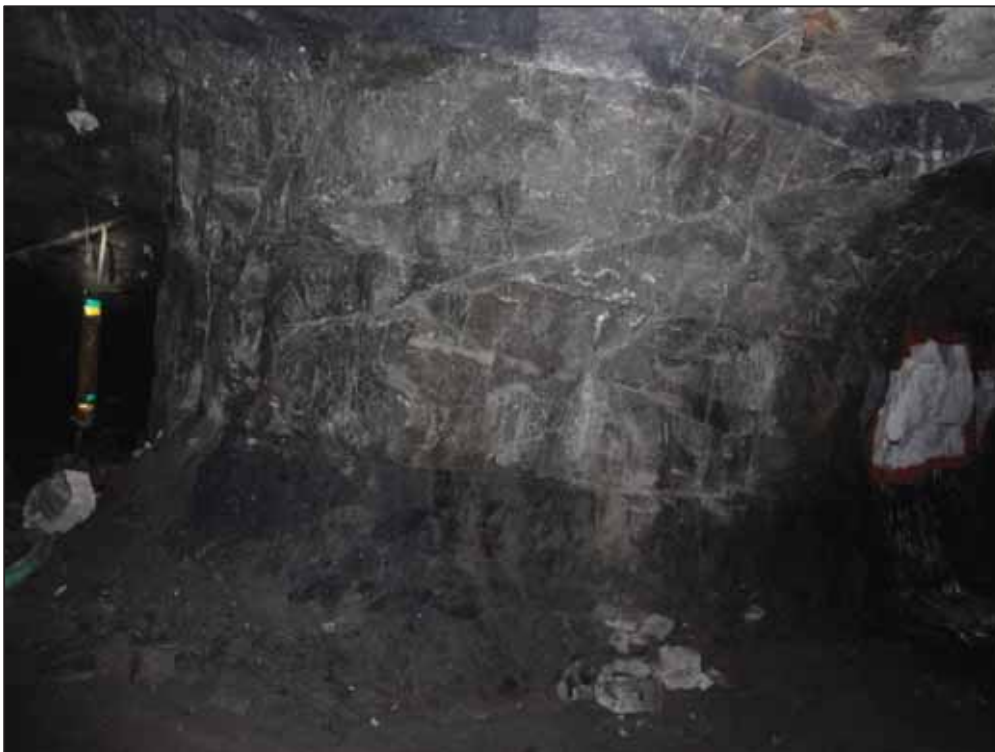
Figure 23: Jointing and layering observed in pillar (Mine 5)
