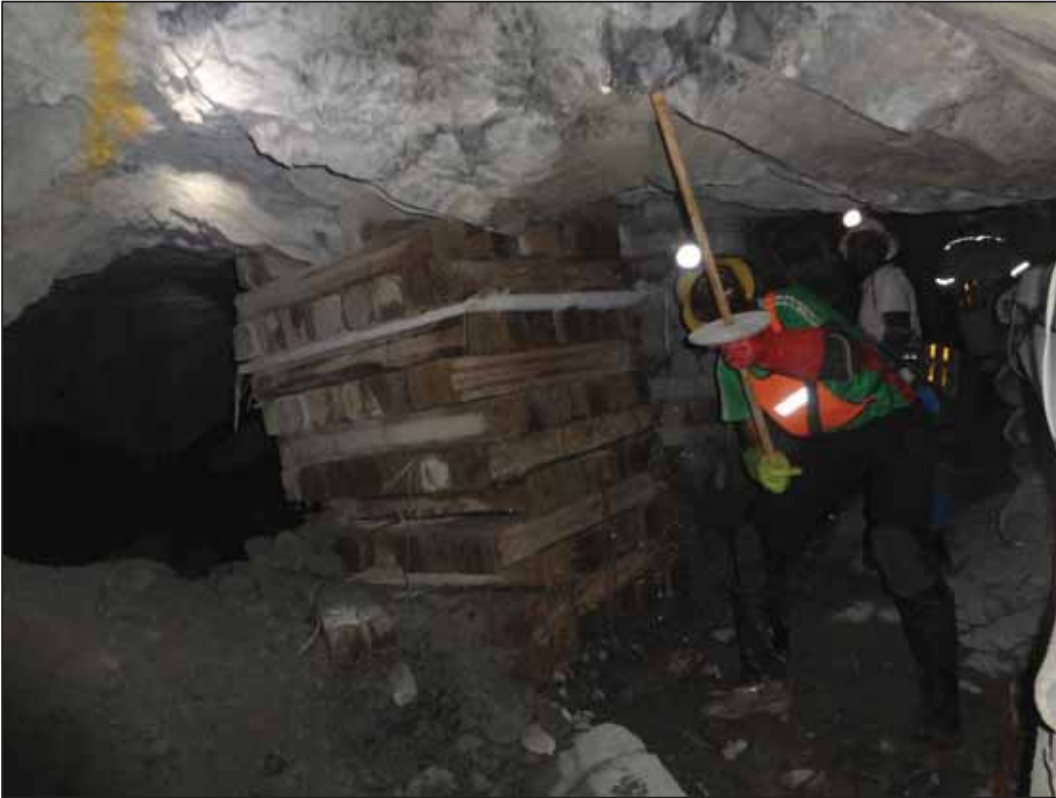
Figure 67: Typical conventional stope where height of excavation is less than 2m (Mine 8)
