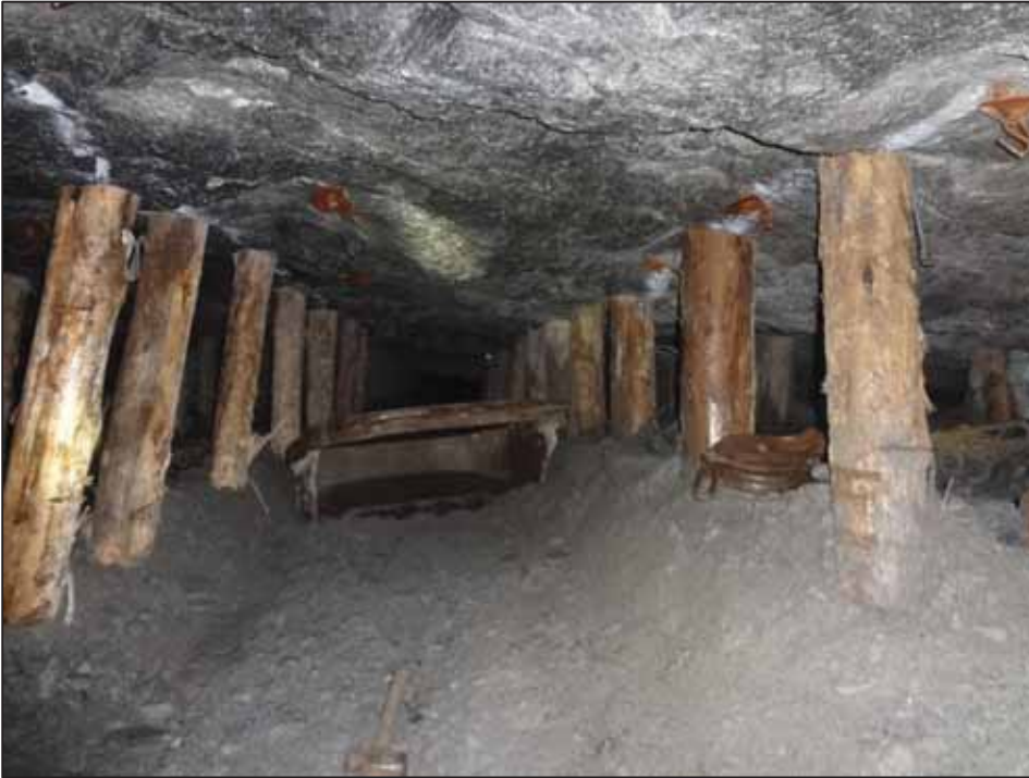
Figure 27: Typical conventional stope where height of excavation is less than 2m (Mine 8)
