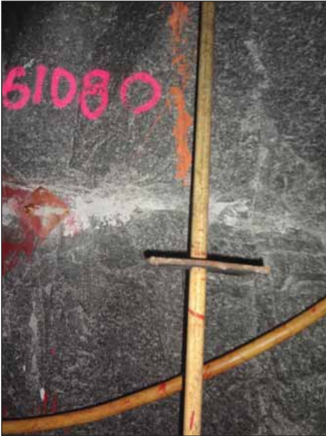
Figure 21: 3m long Fiberglass pinch bar used at a development end at Mine 8
