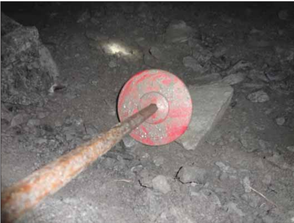
Figure 18: Incorrect usage of a drill steel gasket which does not fit tightly onto the pinch bar (Mine 6)
