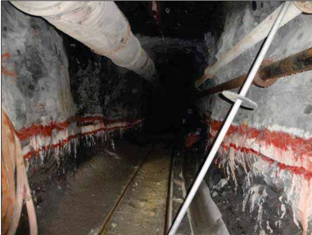
Figure 65: Pinch bar with mine-made gasket - possibly conveyor belt (Mining House D)
