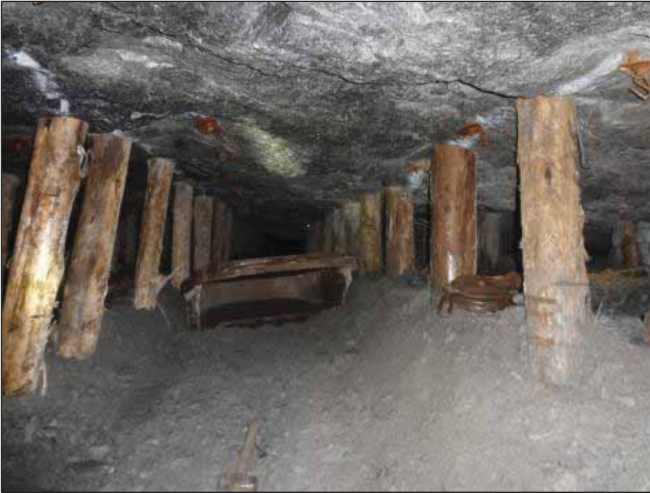
Figure 42: Typical conventional platinum stope where height of excavation is less than 2m (Mine 8)
