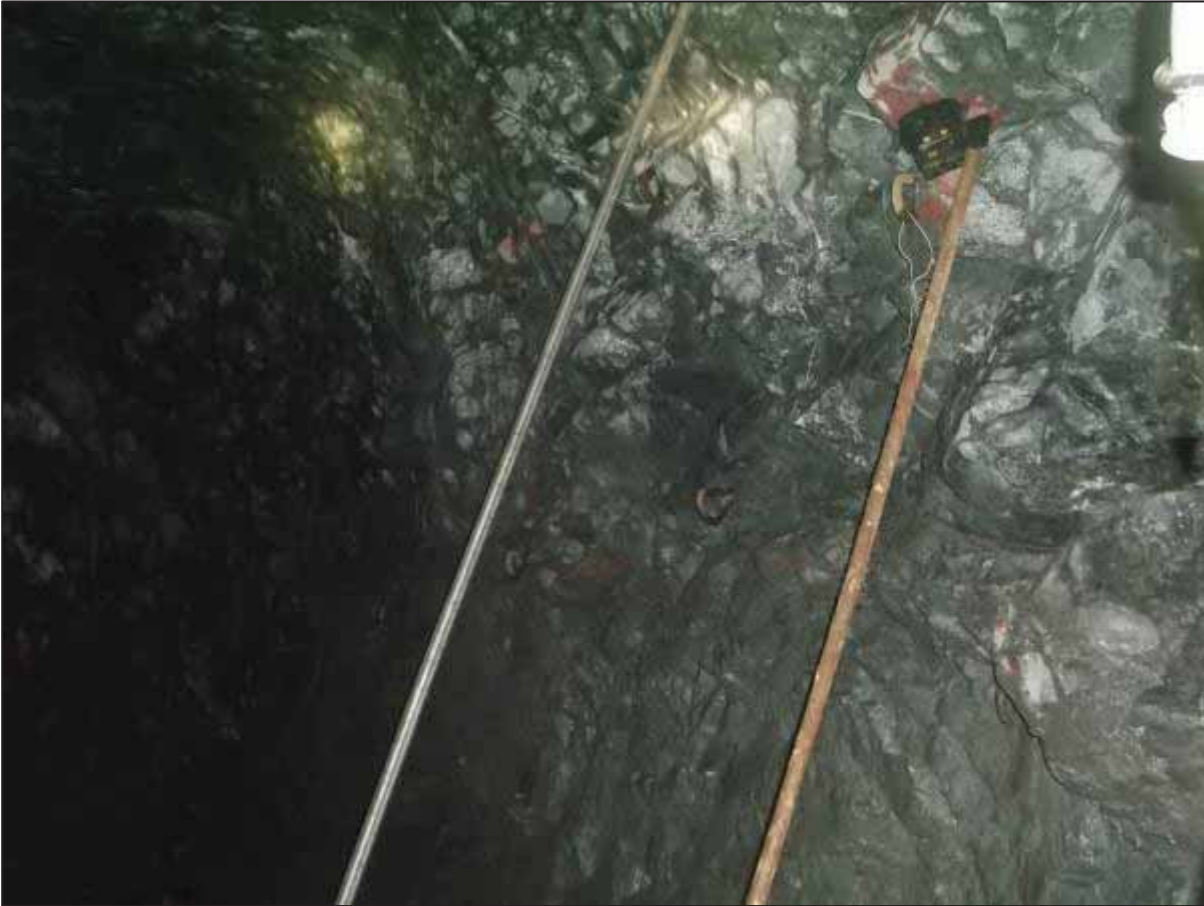
Figure 70: Long Pinch bar ready to be used in a development end for barring with no gasket fitted on. The pole alongside the pinch bar is used to extend the GDI to test for gases at the top of excavations (Mine 7)
