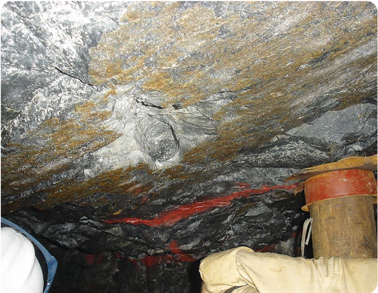
Figure 1: Poor drilling discipline results in sockets in the hangingwall
