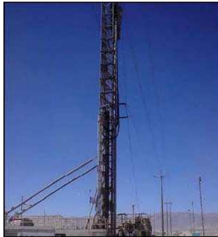
Figure 32: SME in close proximity to overhead power lines
