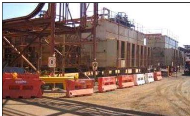
Figure 18: Demarcation of construction site
