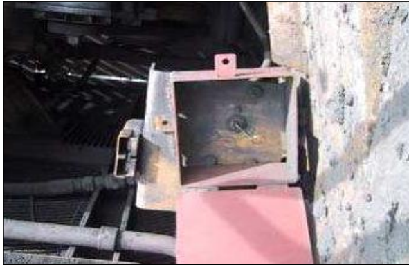
Figure 5: Unacceptable Isolation
