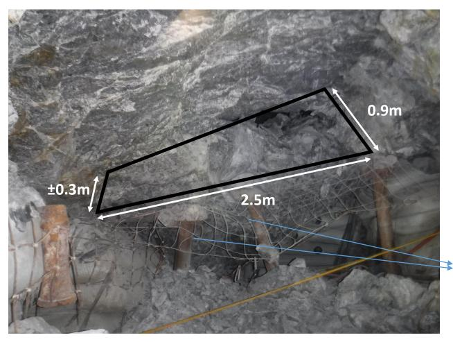
Two props installed to break the span between the backfill
