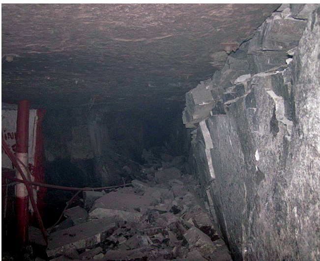
View from South along pillar from 13 West
