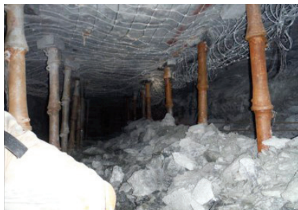
Undercut panels with stoping width 1.8m – RB80 props and steel netting
