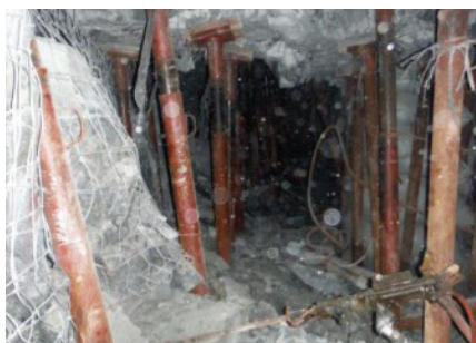
Open cut panels with stoping width >2.5m – Omni props and steel netting
