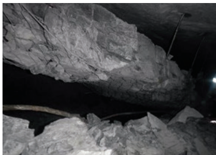
Raise line 1810 S13A centre gully hanging wall was supported with permanent mesh and tendons. Subsequent to the initial breast ledge blast, a significant FOG of 72 tonnes was suspended by the permanent mesh.
