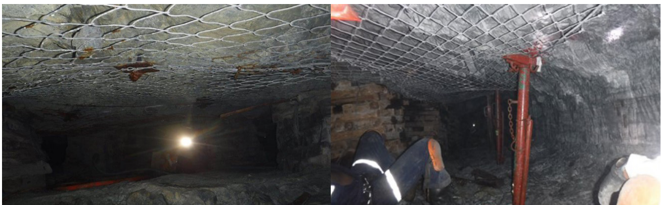
Figure 14: A. Permanent in-stope steel net arresting a seismic induced FOG following a magnitude 2.4 event at 1810 S12 E17 UD3 on 24 May 2022. B. FOG related accidents statistics over a nine-year period.
