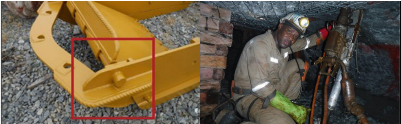
Figure 13: In-stope permanent netting installed with rock-studs and bigger washers and temporary mechanical jacks in a panel at Masimong Mine
