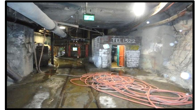
28 Level towards the fridge plant – dusty station areas washed daily
