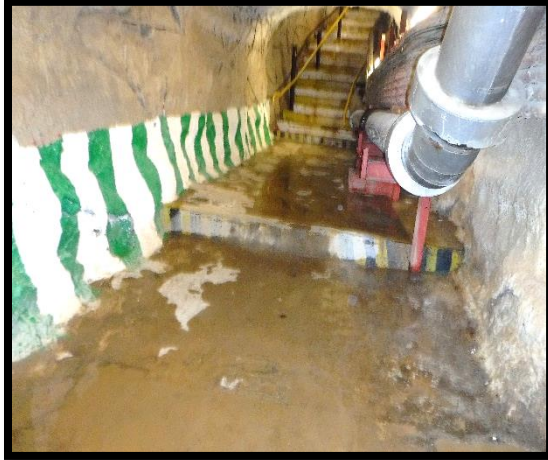
Travel way to Tertiary Shaft washed down
