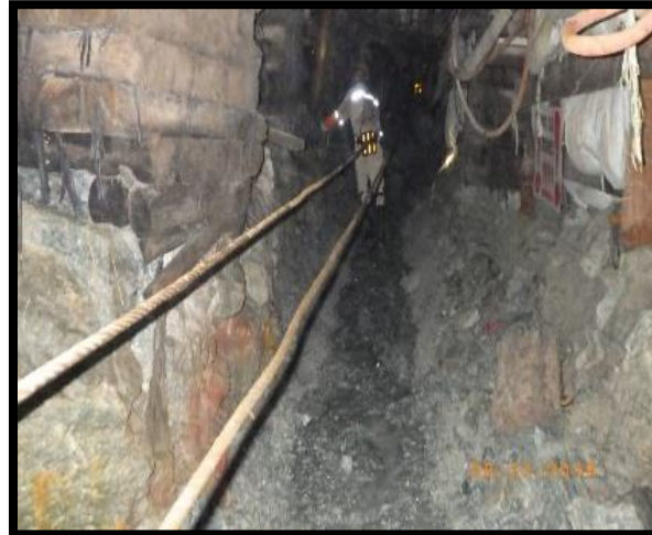
3E Gully – watered down using an open-ended hose
