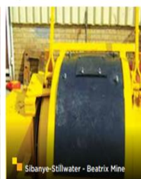
Scraper winch cover after
