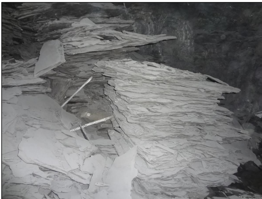
Figure 43: Large FOG in old area in the section. Picture taken to show the laminated nature of Shale and Coal in the roof
