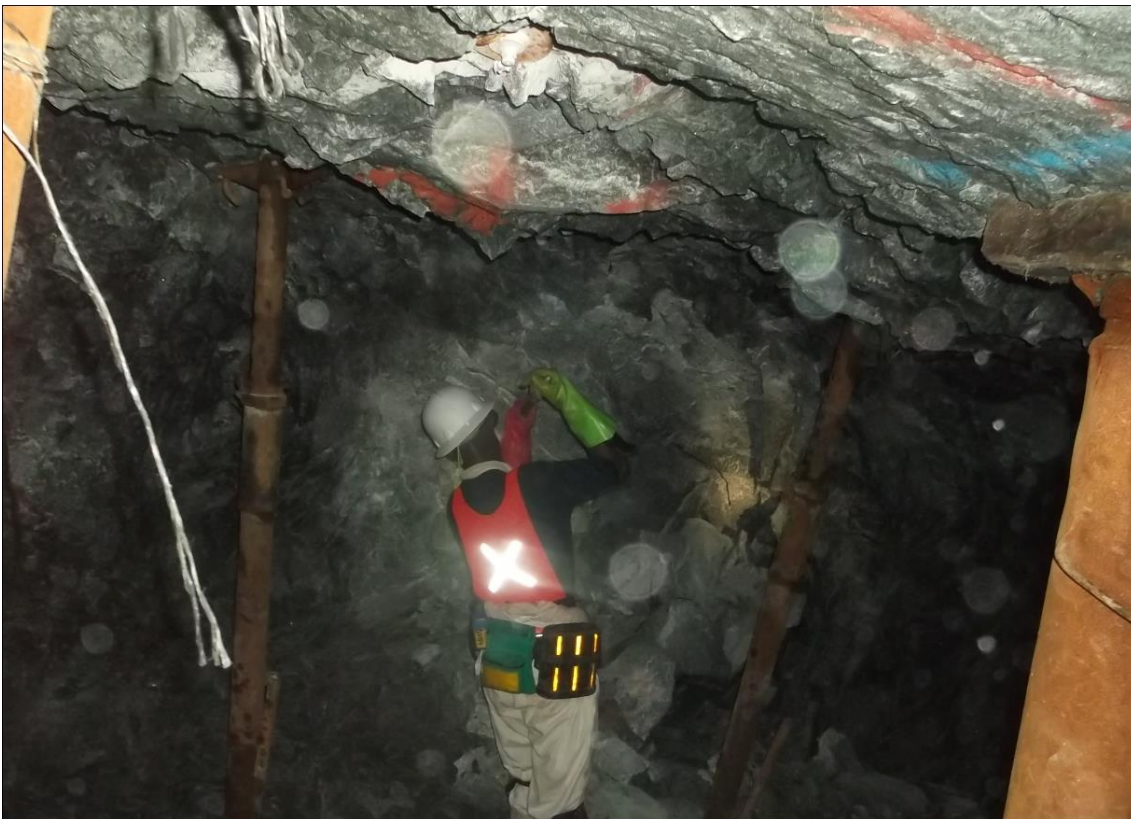
Figure 87: Barring at the face
