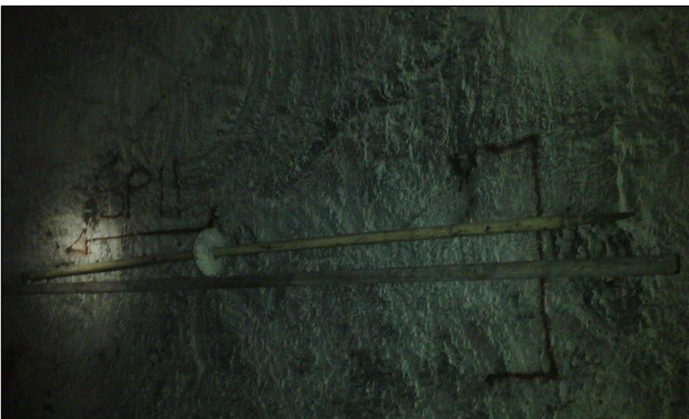
Figure 38: More barring equipment in section
