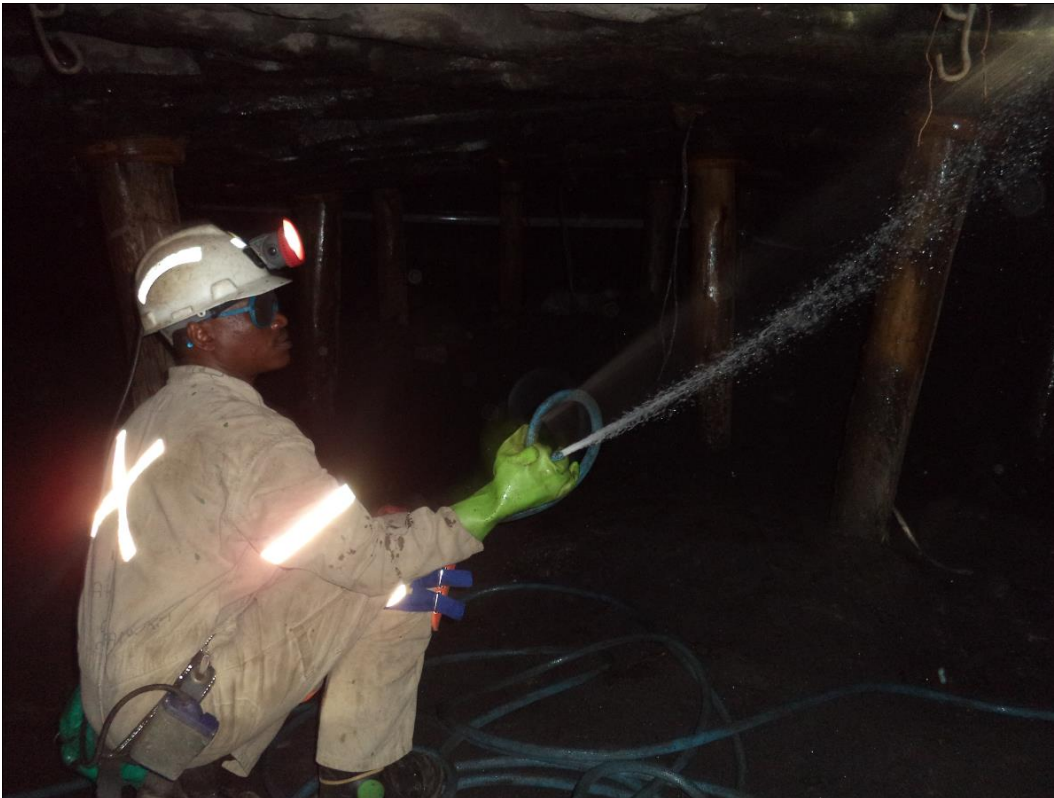
Figure 62: Watering down prior to barring
