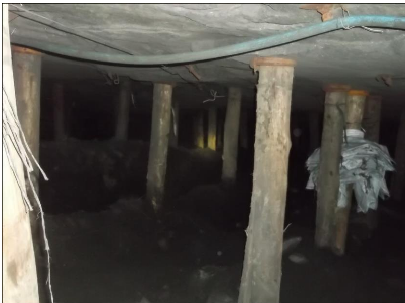
Figure 83: Smooth HW condition
