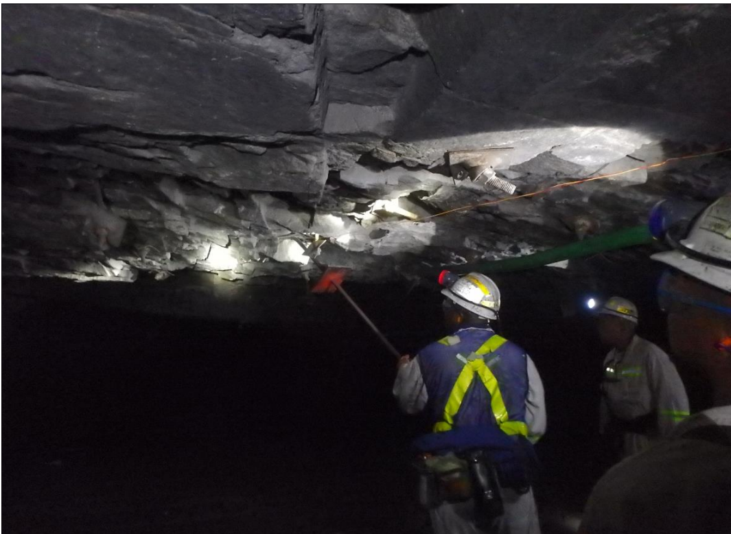
Figure 73: Barring blocky hanging wall
