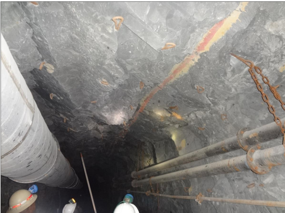
Figure 27: HW in tunnel
