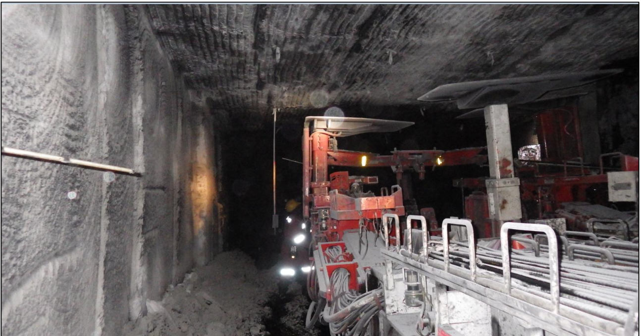
Figure 46: Good Roof conditions and good pillar cutting
