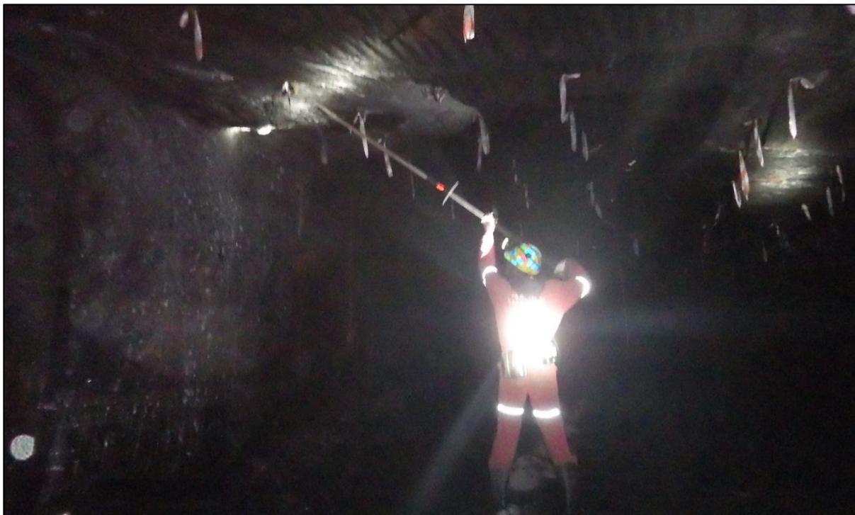
Figure 53: Barring being completed
