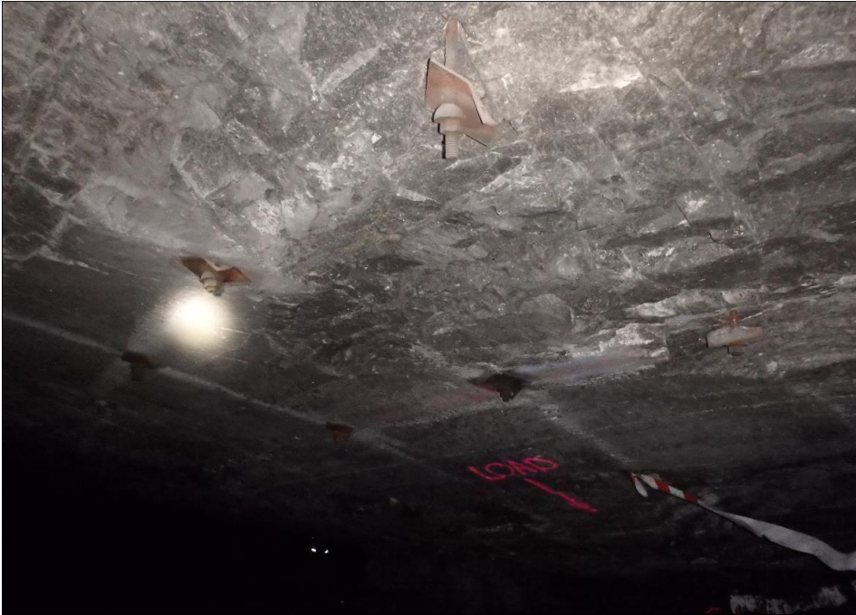
Figure 72: Blocky HW conditions
