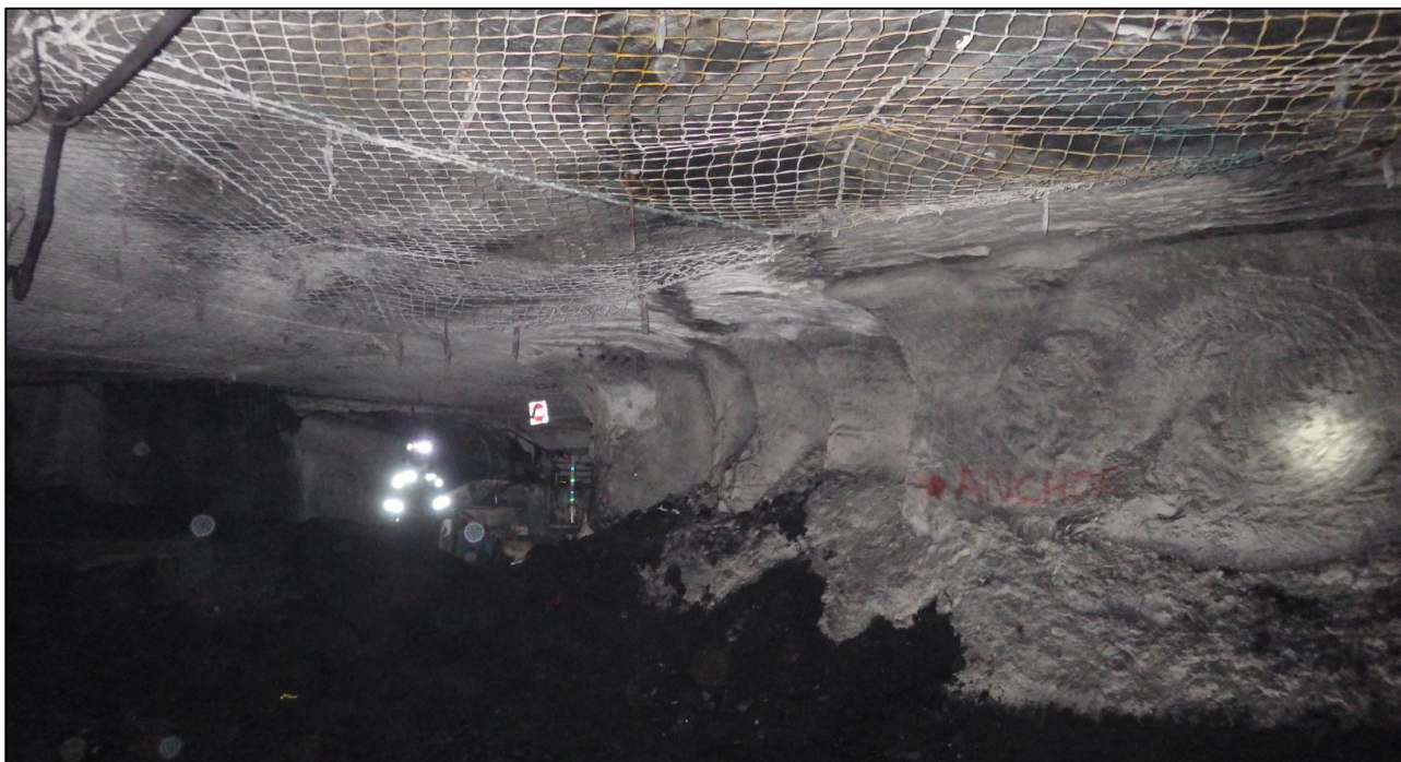
Figure 55: Smooth roof conditions with installed nets
