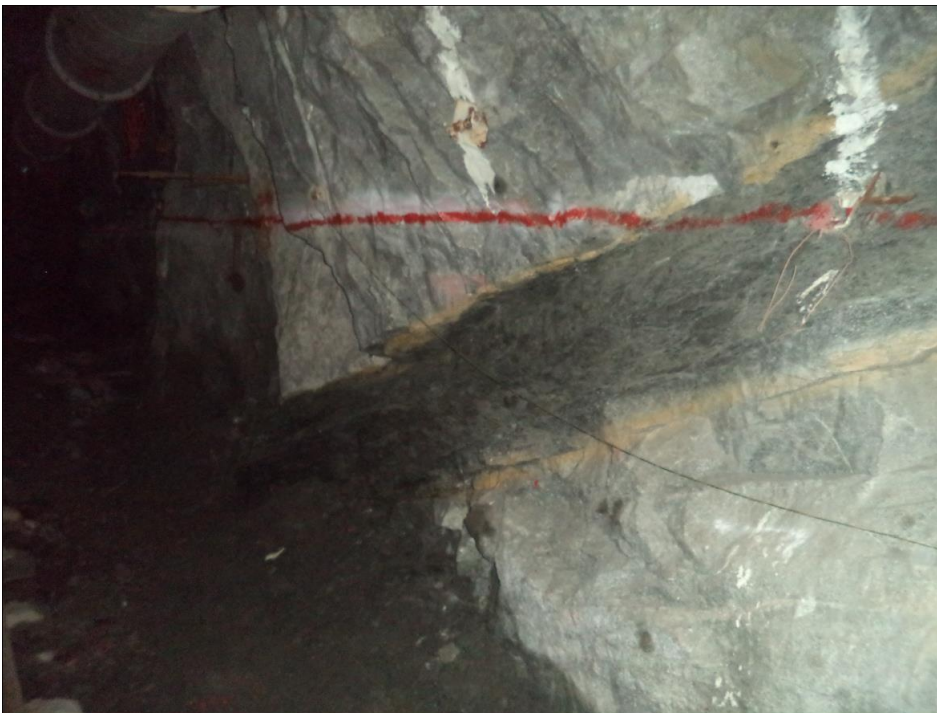
Figure 69: Dyke in Sidewall
