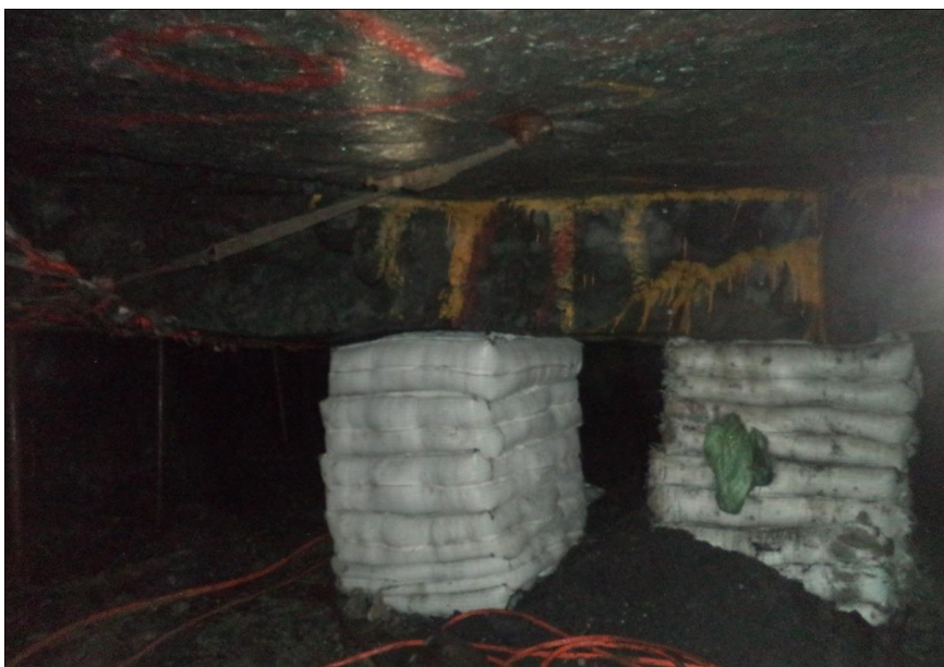
Figure 60: Large Brow supported with Grout Packs
