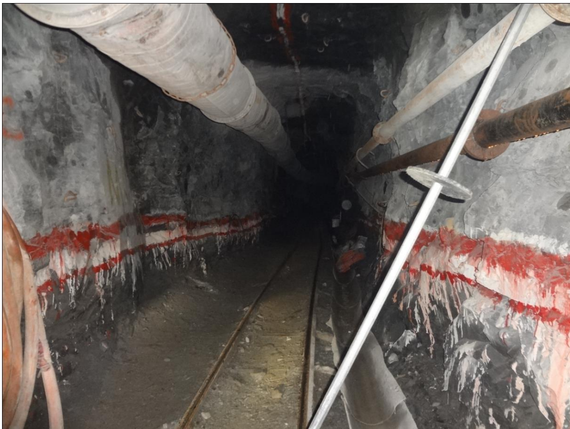
Figure 34: Sidewall and Hanging Wall condition
