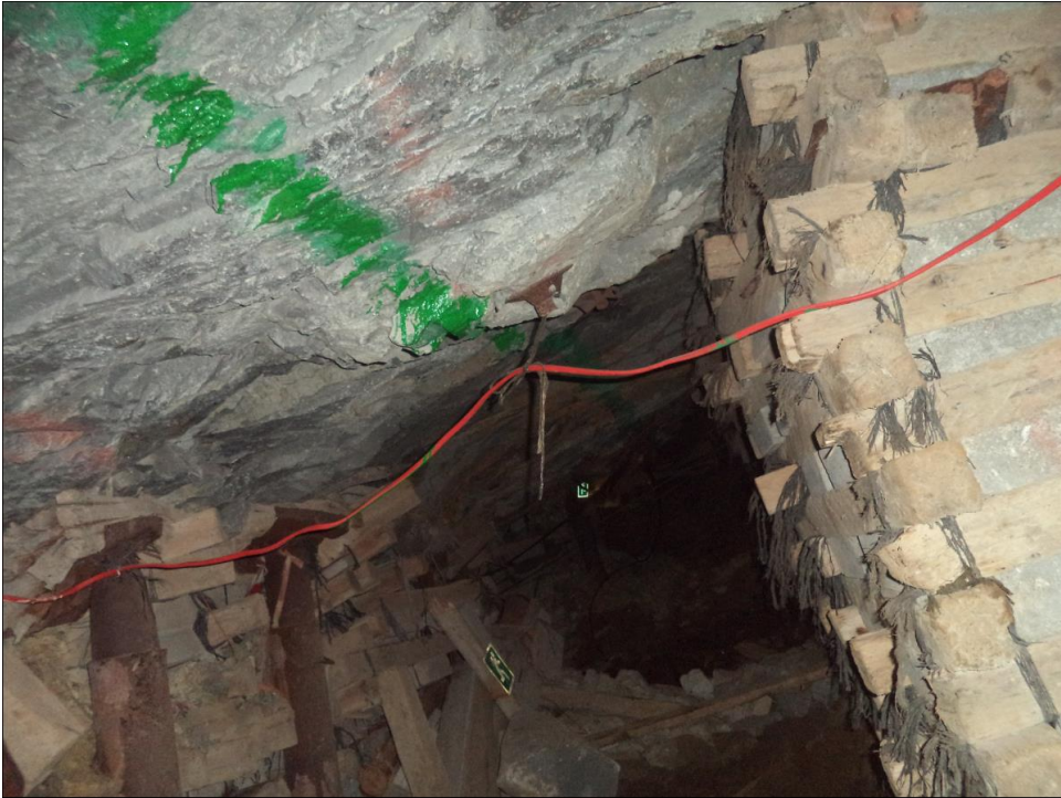
Figure 77: Gully HW condition
