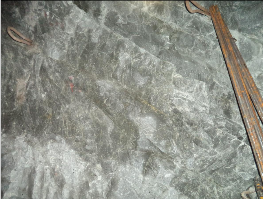
Figure 75: Jointing in Sidewall
