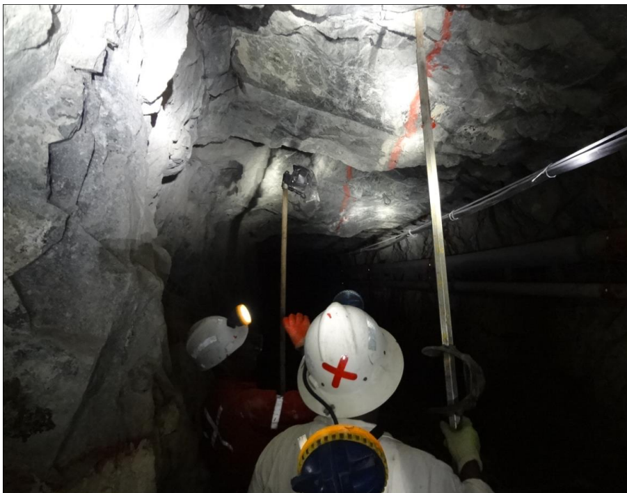
Figure 7: XC Sidewall and HW condition
