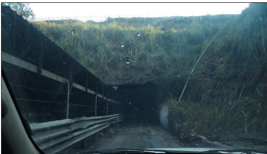
Figure 52: Decline/ Portal entrance
