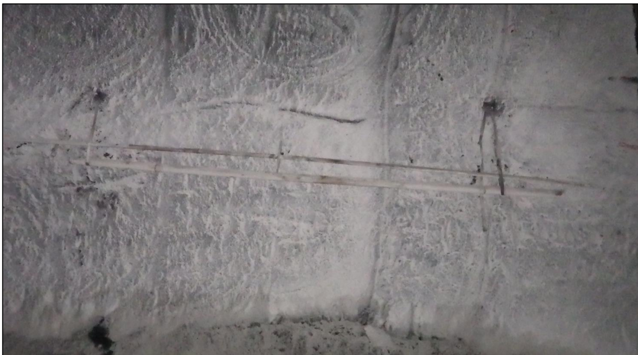
Figure 47: Coal Barring Equipment
