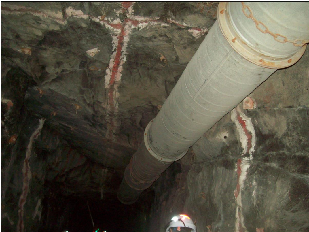
Figure 5: Condition of XC
