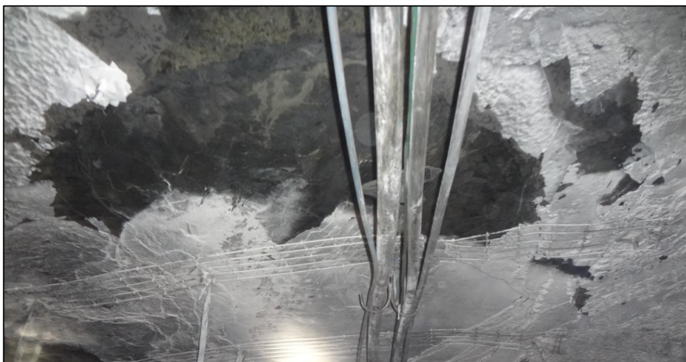
Figure 41: Areas of the roof where barring was completed
