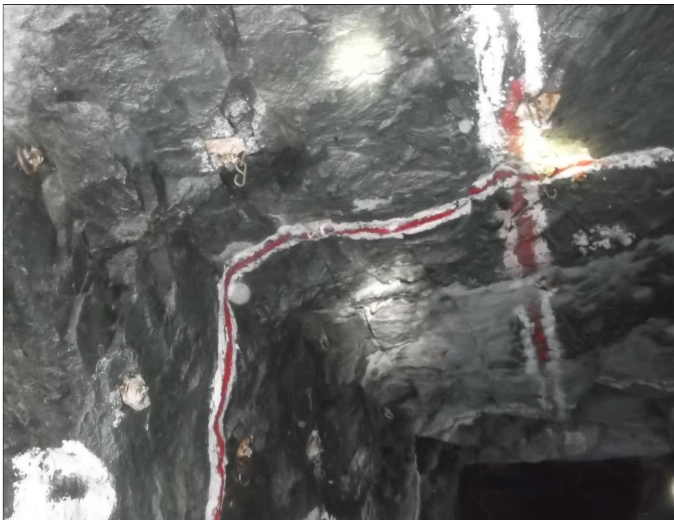
Figure 84: Jointed HW condition
