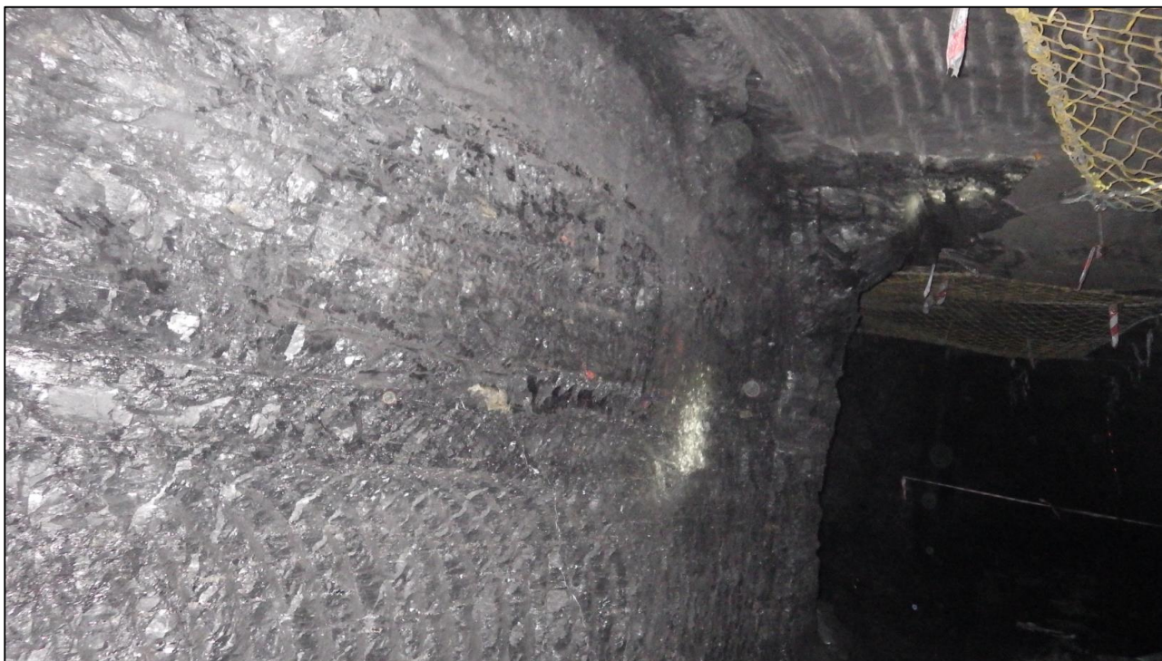
Figure 54: Good Pillar conditions and nets tensioned against the roof
