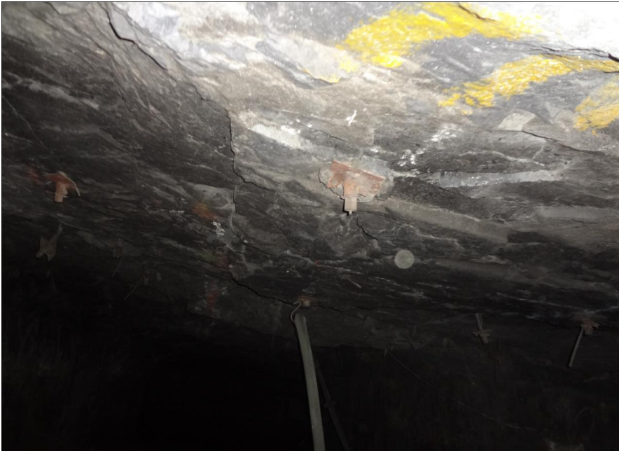
Figure 12: Relatively smooth HW
