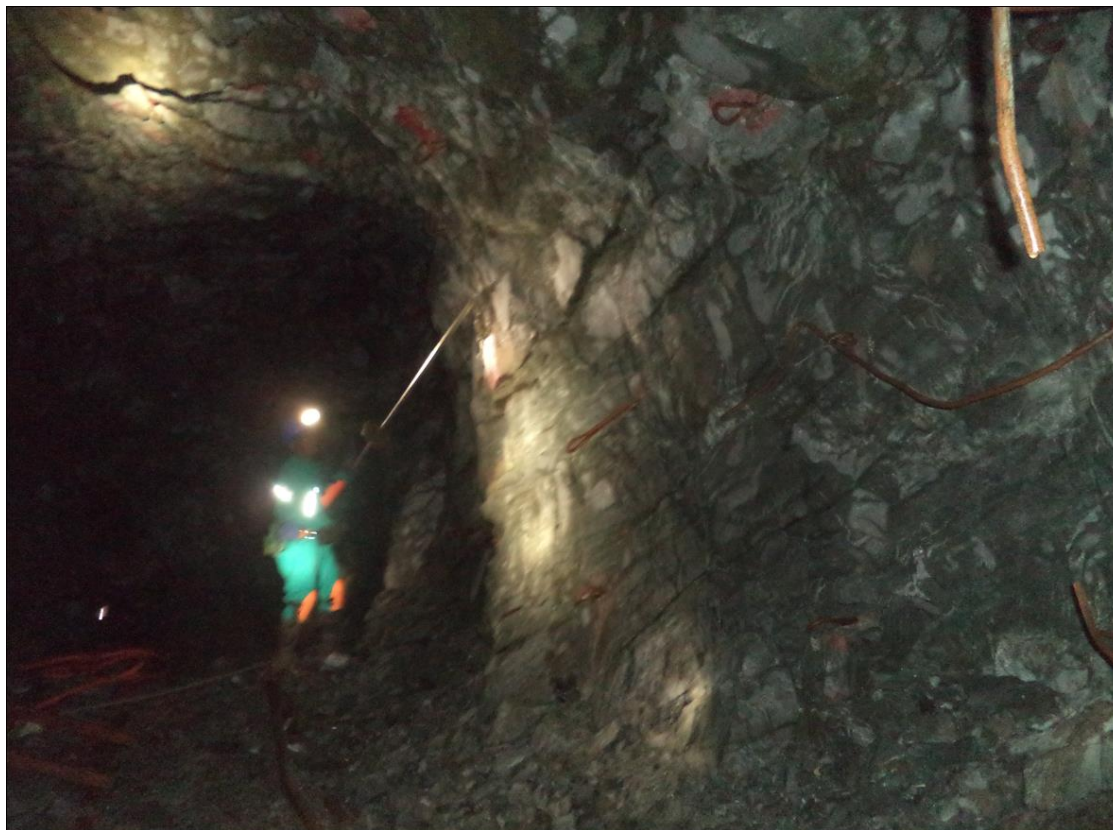
Figure 76: Barring in high excavations
