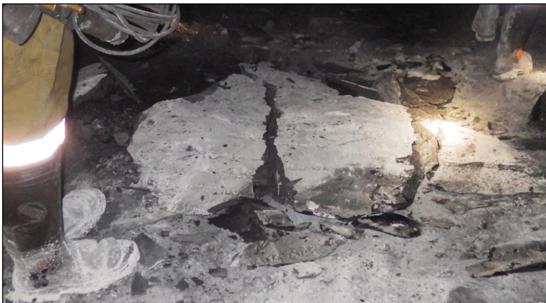
Figure 51: Size of rocks barred down
