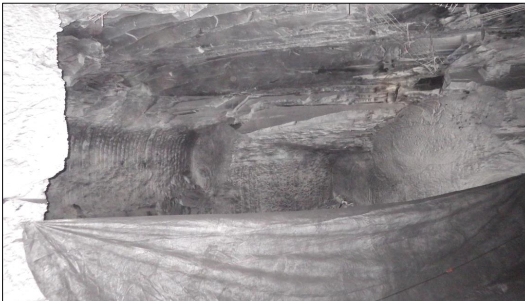
Figure 50: Roof laminations
