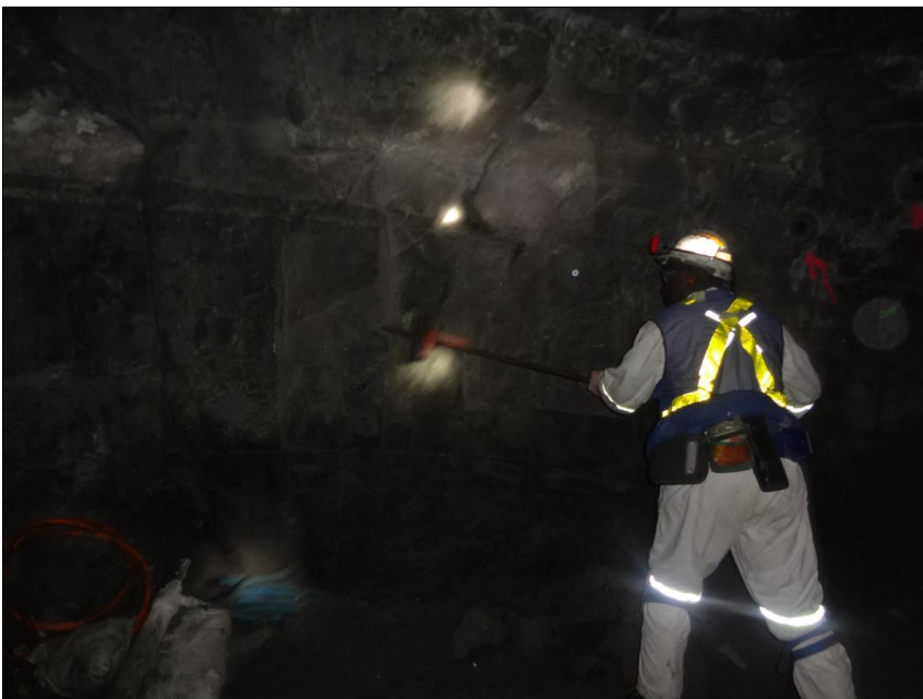
Figure 11: Barring of pillar sides
